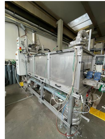
REC AUGER reactor
